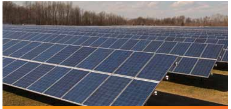
PROJECT NAME PARADISE SOLAR ENERGY CENTER Size: 6.2 MW Location: Paulsboro, New Jersey Project Type: Utility Number of Modules: 26,224 Installer/Partner: American Capital Energy and Nextera Energy Resources
